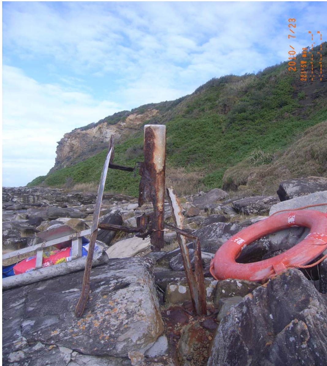
The original 1994 post or what was left of it after it finally rusted away in July 2010
